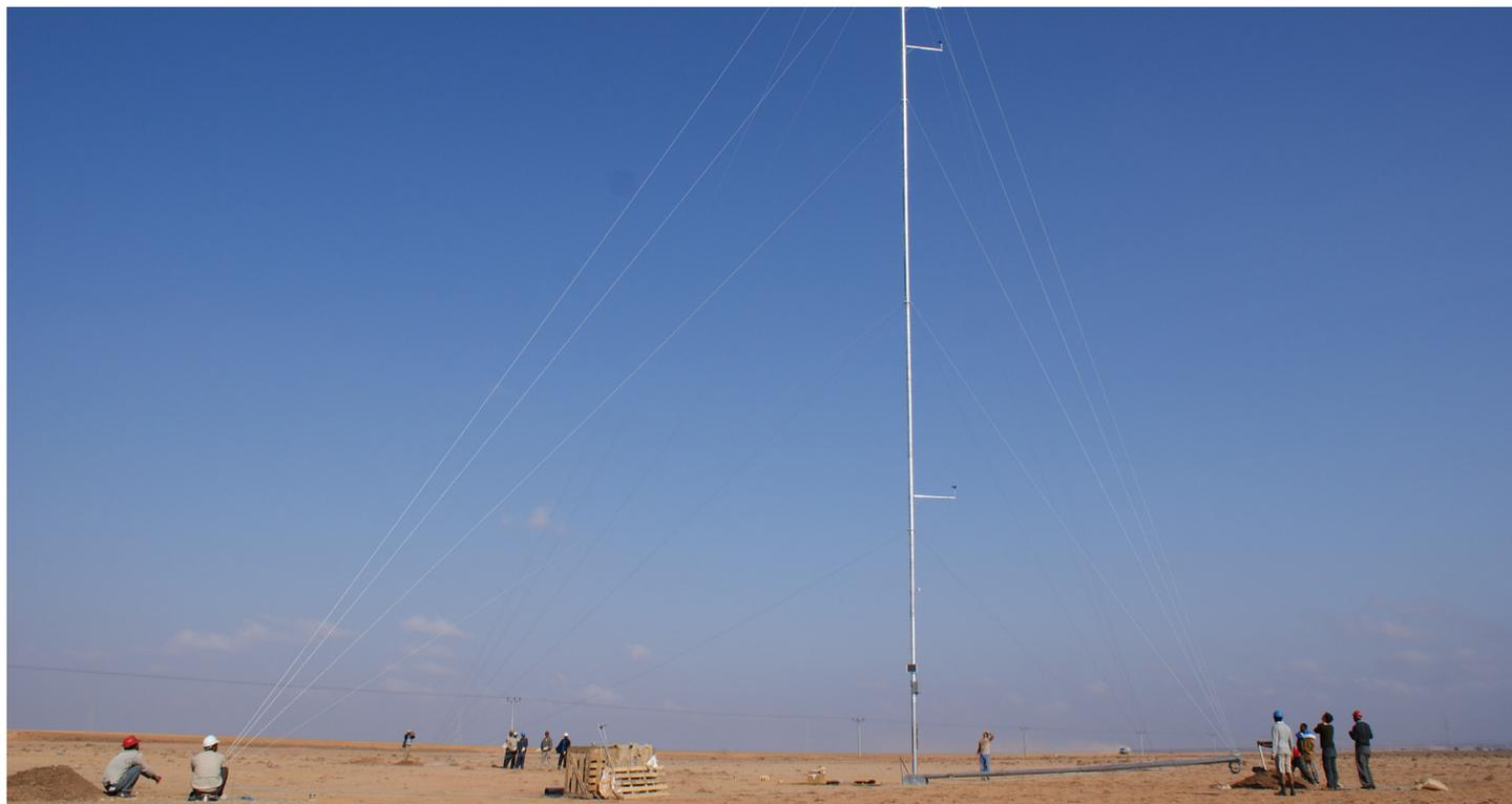
Ethiopia's first 40 metre wind measuring mast being erected in Aysha in January 2010. The certified mast was made possible through funds and technical know-how transfer from the PPP
